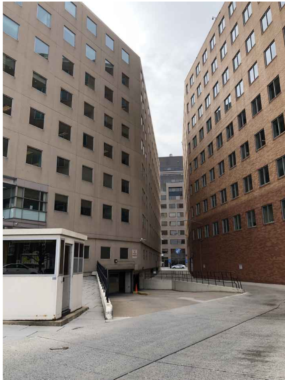
1. Public Alley, Looking South
