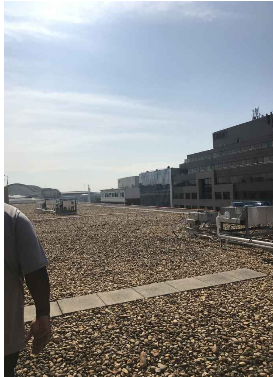
2. SE View from Roof
